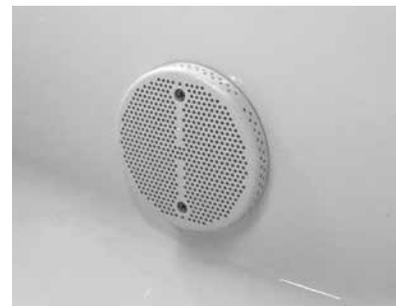
For soakers and air baths, the water is drawn in through an intake such as the one shown, flows through the inline heater and is reintroduced into the bath through an output that has the same appearance.
